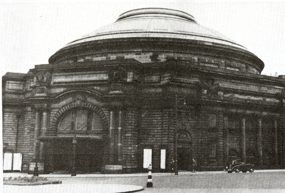
THE USHER HALL. It is hoped the long-promised renovations will include acoustic improvements and civilised refreshment services.
